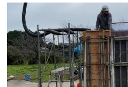
Pic.1 Placing point
